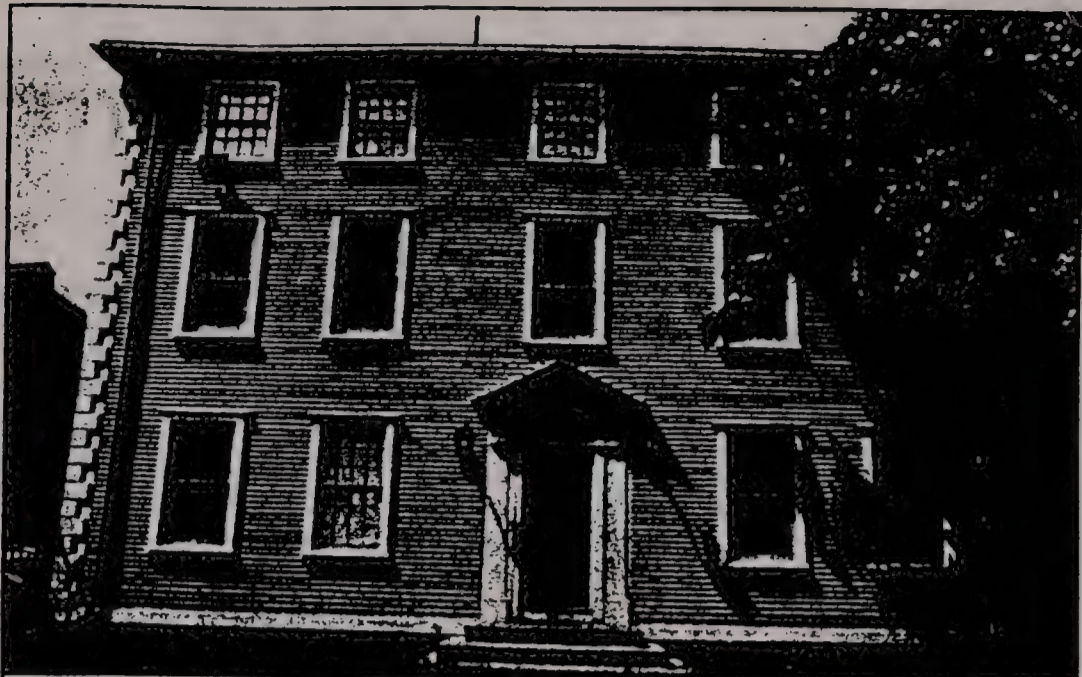
To restore the original Federal-style exterior, owner James Adams had to strip off a one-storey commercial appendage and replace most of the woodwork.
